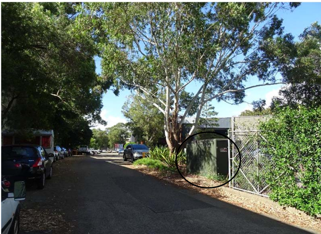
Figure 3: View south along driveway from Bourke Street, with the substation proposed to be relocated circled
